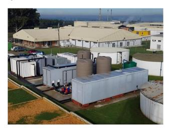
In F2017, County Fair partnered with Proxa to develop a reverse osmosis water treatment plant for the second largest poultry processing facility at Astral, County Fair Hocroft. The water treatment plant utilises Proxa's Aquamobile ultrafiltration and reverse osmosis technologies to provide County Fair with potable water for reuse in production. The reverse osmosis water treatment plant was commissioned in October 2017.
